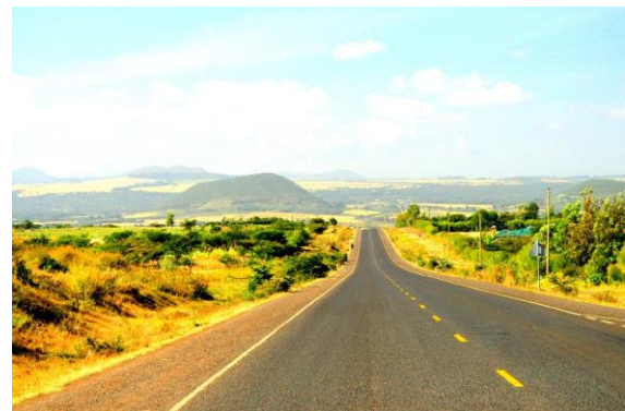
The near completed Isiolo-Moyale road
