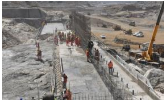
Construction of the GERD (Ethiopian Herald)
